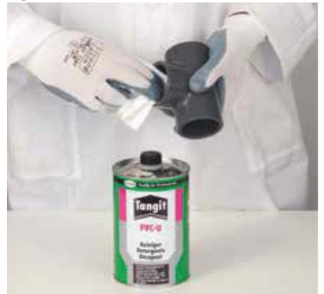
It is advisable to use an applicator/brush of dimension not less than half the diameter of the pipe. The solvent cement must be applied along the entire length of the joining surface of both the pipe and the fitting:
